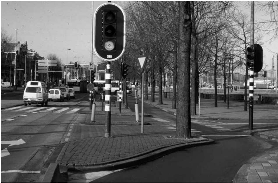
Figure 17. This bike path in Amsterdam swerves to the right several meters to increase cyclist safety when crossing the intersection. The increased distance between the main road and the bike path crossing gives motorists and cyclists more time to see each other and thus avoid collisions. The traffic island with two bollards forces a sharp turning radius for right-turning cars, forcing them to slow down. Cyclists get an advance green light via the two sets of traffic signals shown on the post to the far right, further increasing their speed and safety.
