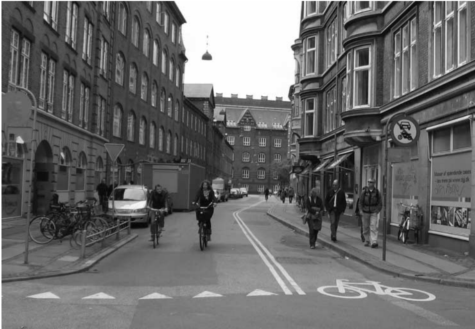
Figure 15. This contra-flow lane in Copenhagen enables cyclists to ride in both directions, while cars are restricted to one direction. The roadway has been deliberately narrowed through the provision of bike parking. In effect, these modifications have turned it into a bicycling street, where cyclists outnumber motorists.
